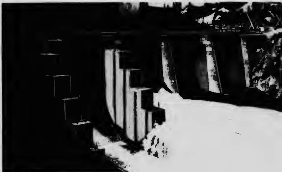
Stave Lake Development. Downstream face of dam.
